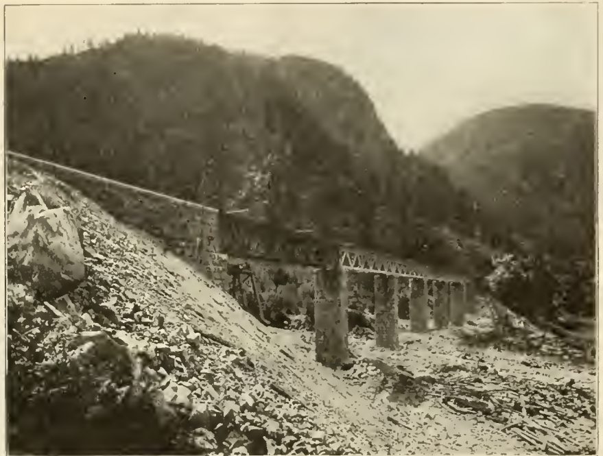
WHITE'S CREEK BRIDGE, B. C., ON THE CANADIAN PACIFIC.
